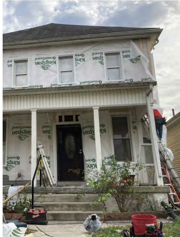
Builders rehabbing a home for Healthy Homes in South Linden.
