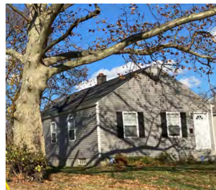
COCIC cleared the title to this parcel. The City Land Bank then sold the property to a small local investor who rehabbed the North Linden home. It is currently a rental.
